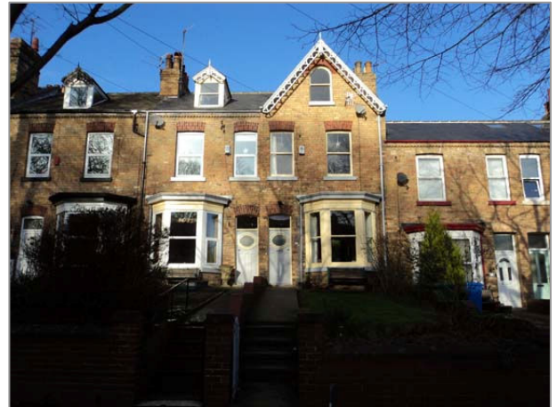
Photo 36: Traditional terraced housing with bay windows and vertical emphasis to the north of the site
