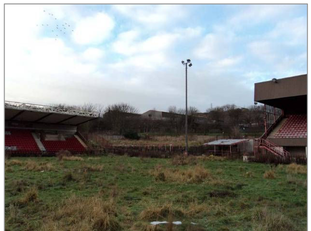
Photo 10: McCain Stadium – Northwest terrace
