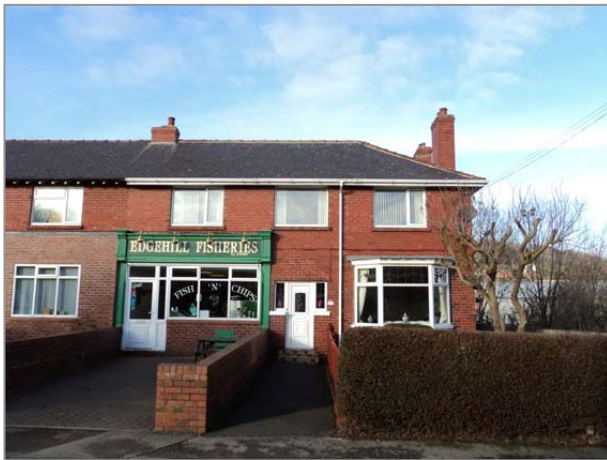
Photo 37: Properties adjacent to the undeveloped ground off Hinderwell Road
