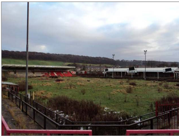
Photo 9: McCain Stadium – Pitch (view southeast from northwest corner terrace)
