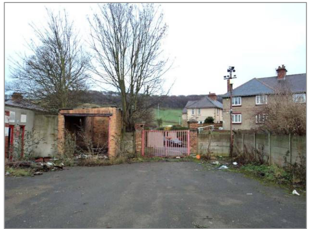
Photo 6: McCain Stadium – Access onto Hinderwell Road
